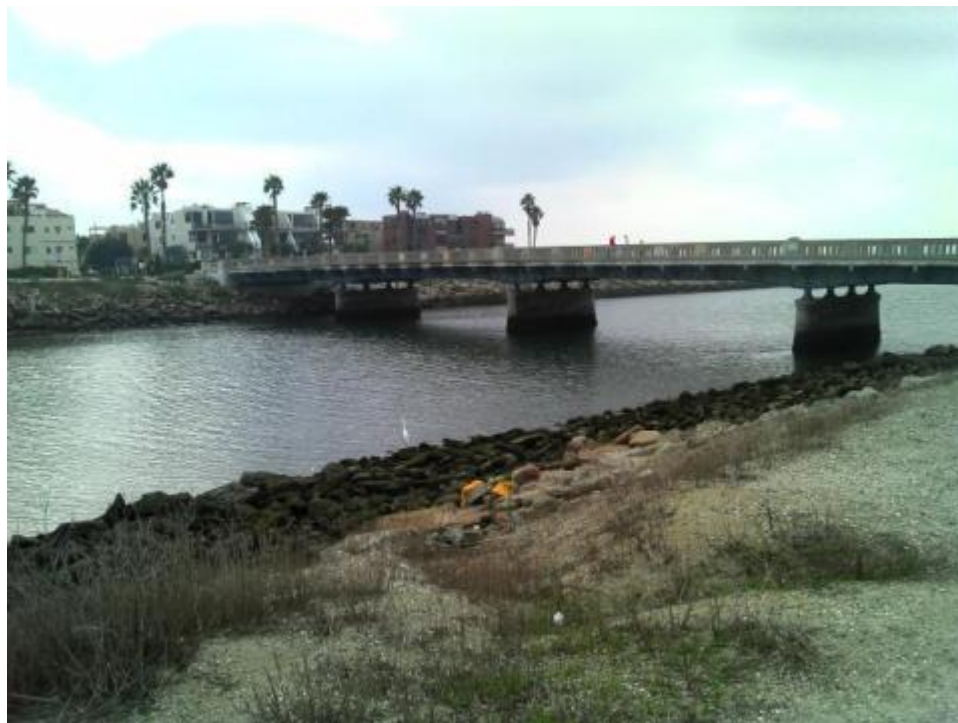
BCE_PAC Ground-Level View
