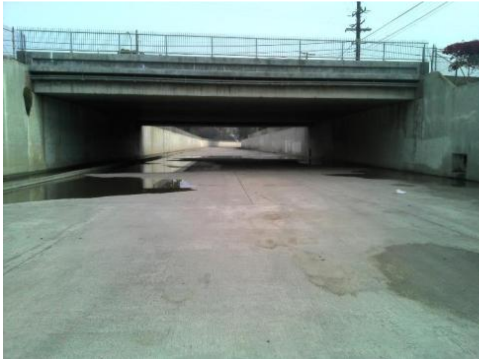
CC_CEN Ground-Level View
