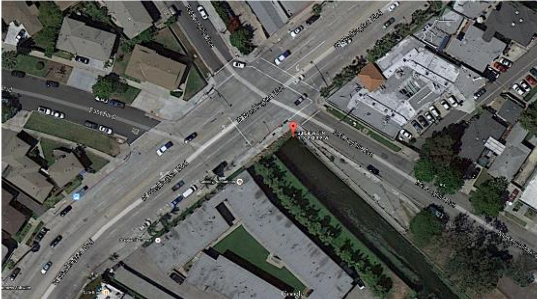
SC_SW_WAS Aerial View
