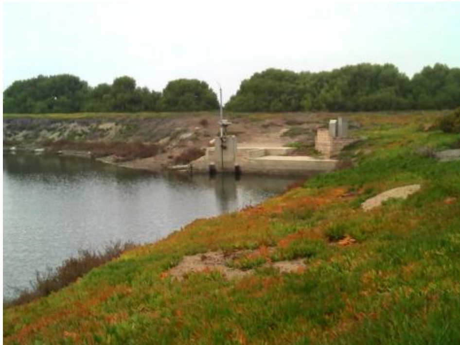
DRL_BCE Ground-Level View
