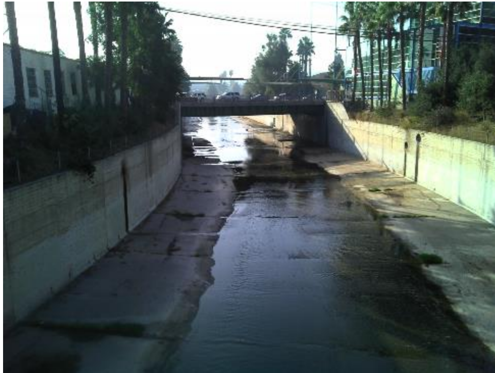
BC_01_WAS Ground-Level View
