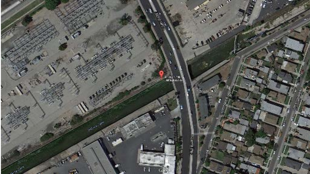
BC_SW_FAI Aerial View
