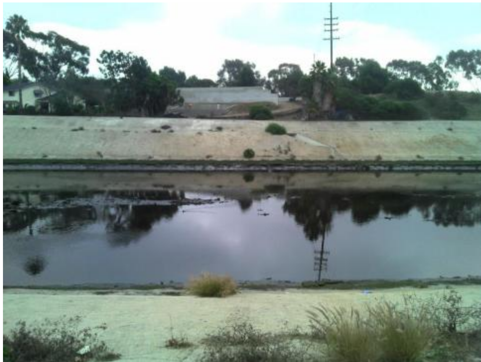
BCE_MCC Ground-Level View
